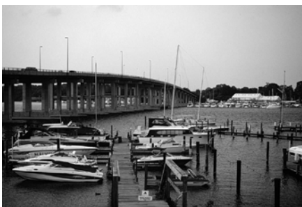
MD2 bridge over South River
